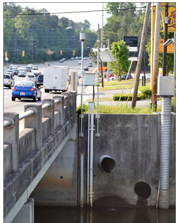
The GIL-B Monitoring Station
